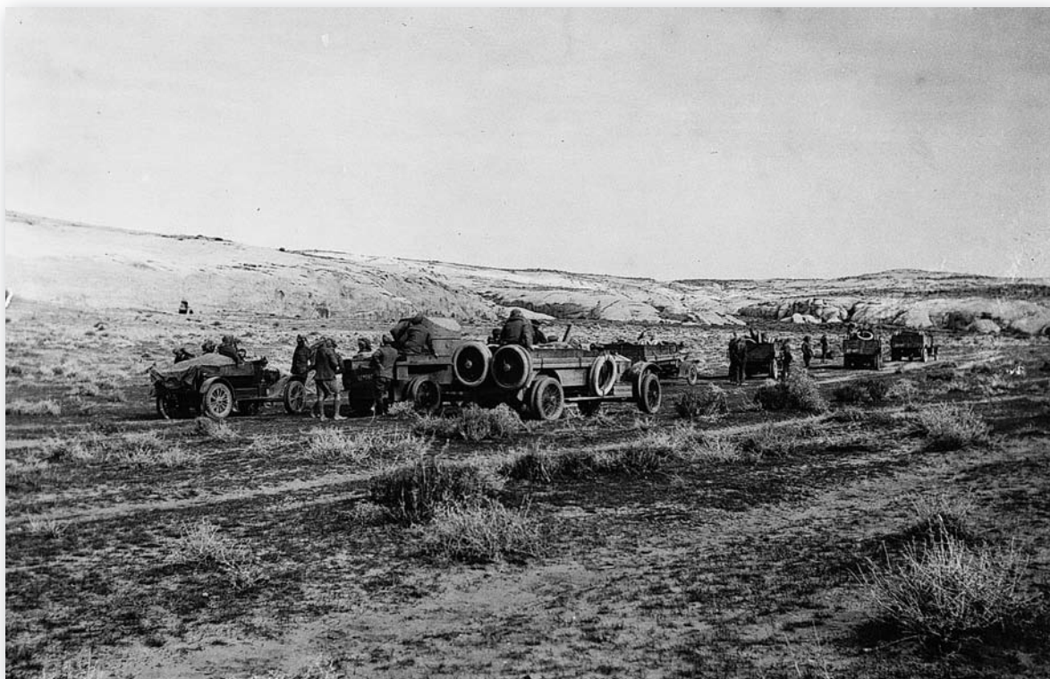
Ford cars, Talbot cars and Rolls-Royce armoured cars at Abu al-Lissan in 1918. The firepower of these mobile units aided both tribesmen and the Arab Regular Army in their attacks. Some of the Talbot cars were mounted with 10-pdr guns while the Rolls-Royce cars carried Vickers machine guns. The numerous spare tyres carried here speak volumes about the terrain. Such units pioneered methods of desert travel that were later used in World War II. (IWM Q59529)
