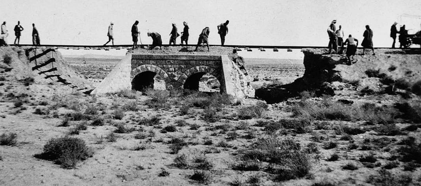
A Turkish repair gang working on a damaged section of the Hejaz line. It is believed that Lawrence, rather cheekily, took this photograph having caused the initial damage. The Ottoman Army expended large resources in keeping the line open during the war. (IWM Q60166).
